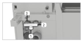
1 = 3/4" common water supply line. (cold water up to 30°C [86°F])
